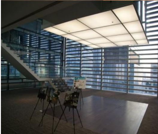
Left: One of Tower C's atriums showing horizontal curtain wall partition
